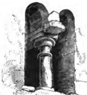
12. Belfry Window of the supposed Saxon character, Wickham, Berkshire.
